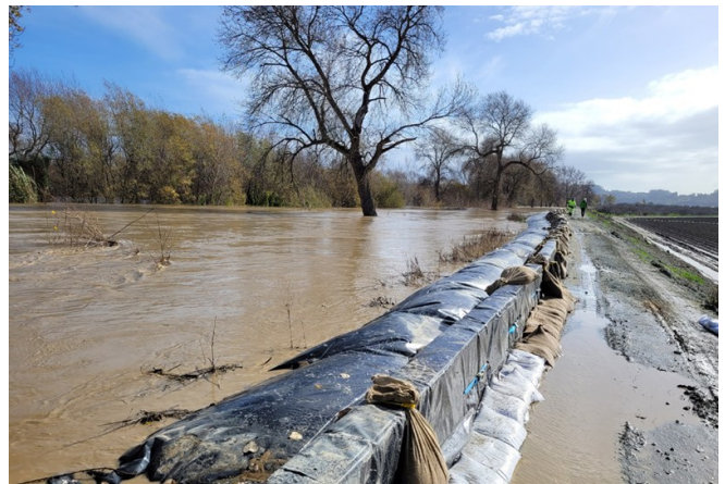
Figure 3. Muscle Wall installed and in action, keeping flood waters from overtopping a levee.
