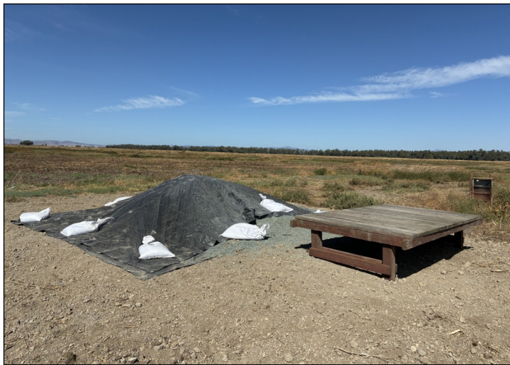
Stockpiled sand near possible problem areas on an exterior levee, ready to be bagged and utilized in an emergency event.
