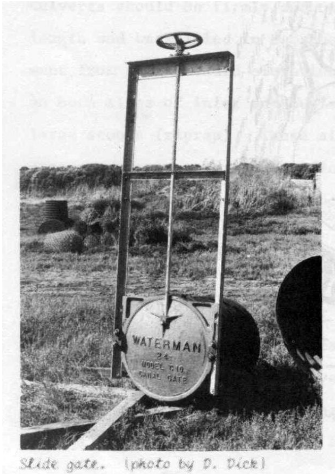
Figure A-8. Slide gate. Photo by D. Dick (Rollins 1981).
