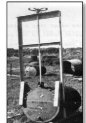
Figure XX. Slide flap gate.
