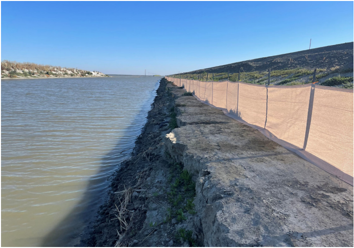
Installed erosion control fencing on the waterside berm
