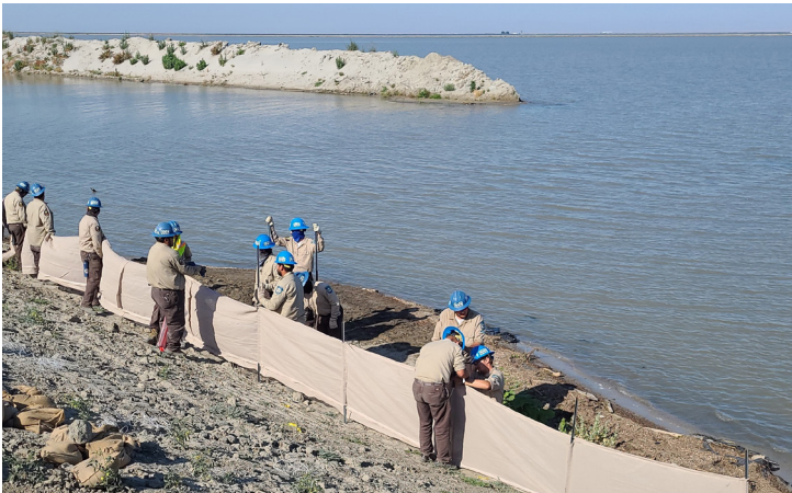
CCC members installing erosion control fencing on the waterside berm
