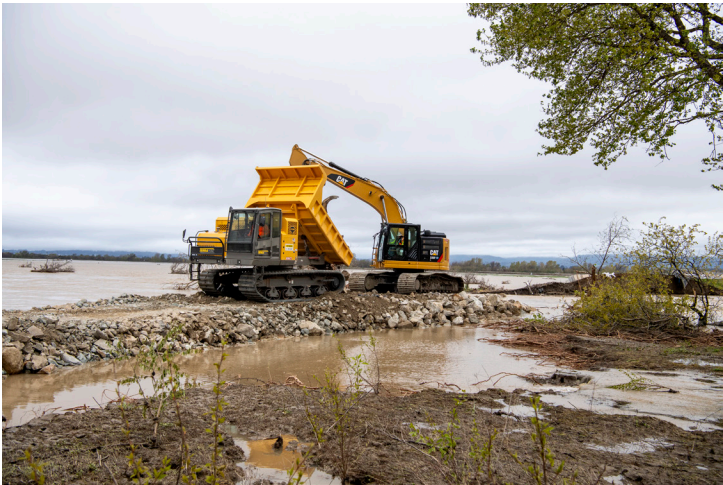
Heavy equipment being used during an advance flood fight
