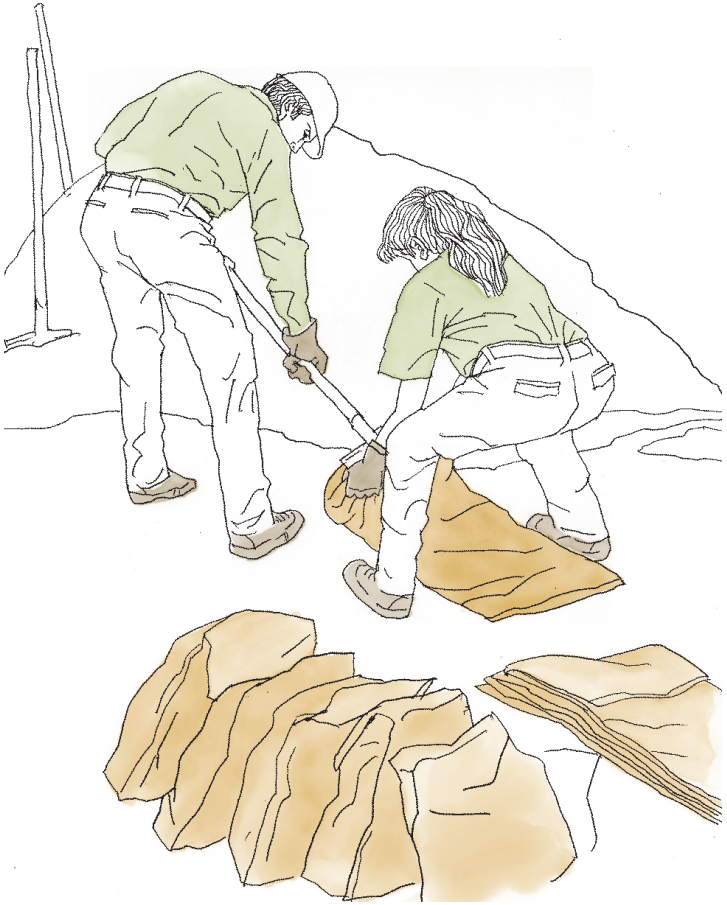
Figure 1: Proper sandbag filling
