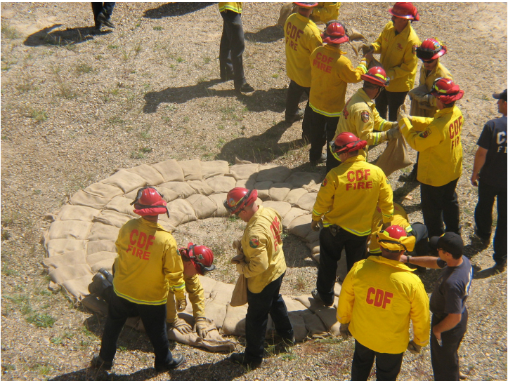
Boil Sack Ring under construction
