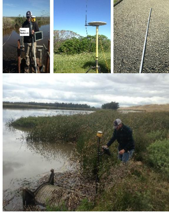
**Figure 3.** Examples of a fixed NGS monument and temporary field benchmark tacs.
